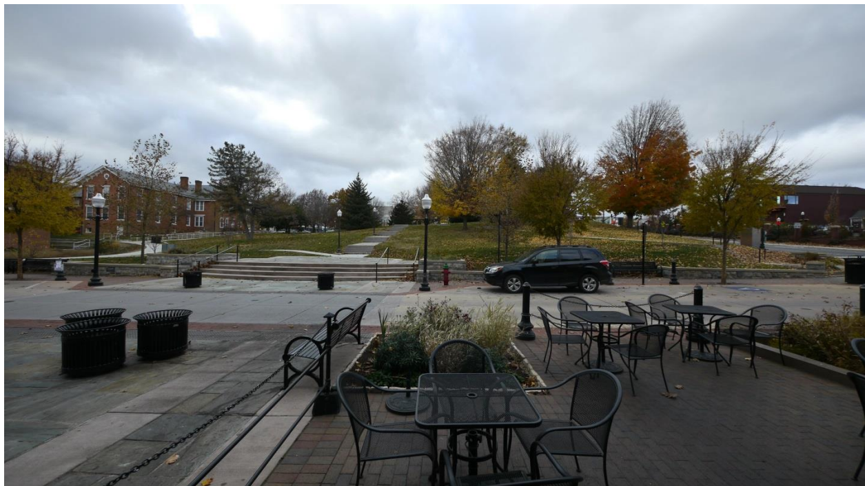
After the conversion: A shared street space where pedestrians and vehicles mingle with a nice open vista in the background.
